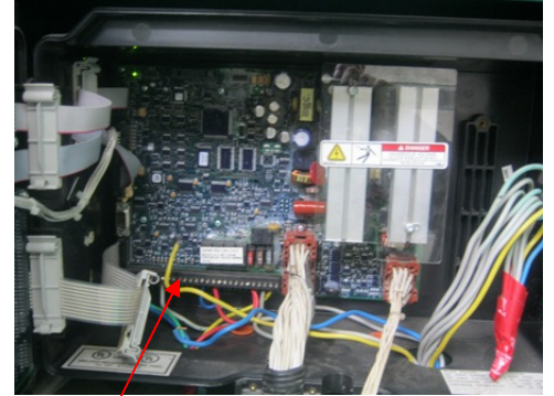
Terminals for remote start / stop on PCC2100
